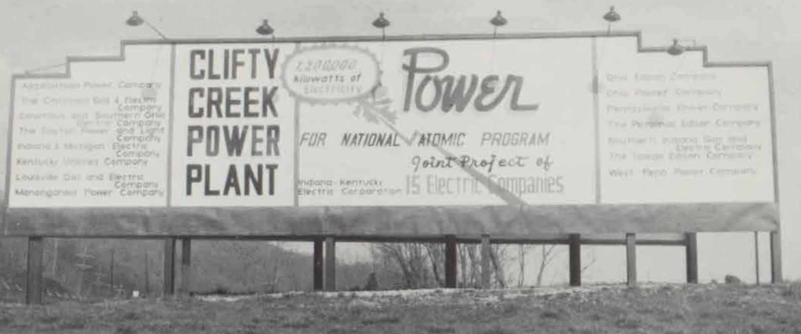
Madison's Clifty Creek Power Plant is an integral part of the National Atomic Program, which is a joint project of 15 electric companies.
